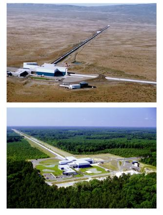
**Figure 2.** Aerial photograph of the LIGO observatories at Hanford, Washington (top) and Livingston, Louisiana (bottom). The lasers and optics are contained in the large corner buildings. From each corner building, evacuated beam tubes extend at right angles for 4 km in each direction (the full length of only one of the arms is seen in each photo); the tubes are covered by the arched, concrete enclosures seen here.
